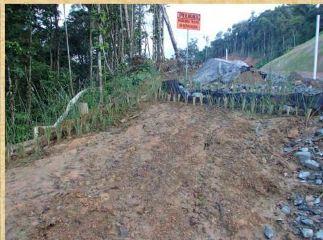
One of the slopes planted well following The Vetiver System did undergo partial failure. This was a fill slope, with gradient about 1.5H:1V. This may be in cause due to poor water
